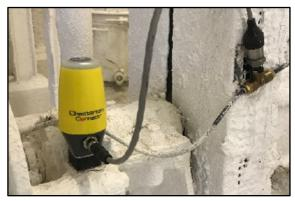
Chesterton Connect attached to slurry pump.
